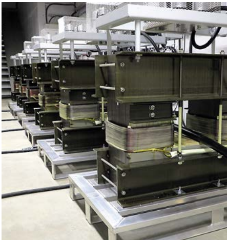
Current transformers in the underground test facility.
